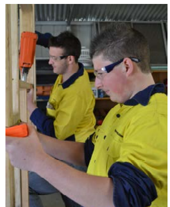
Right: Certificate I in Construction (Doorways 2 Construction) students building a wall frame at Henley High School.
